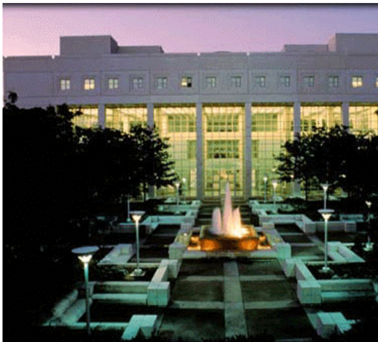
New Library Building, SUNY Albany
